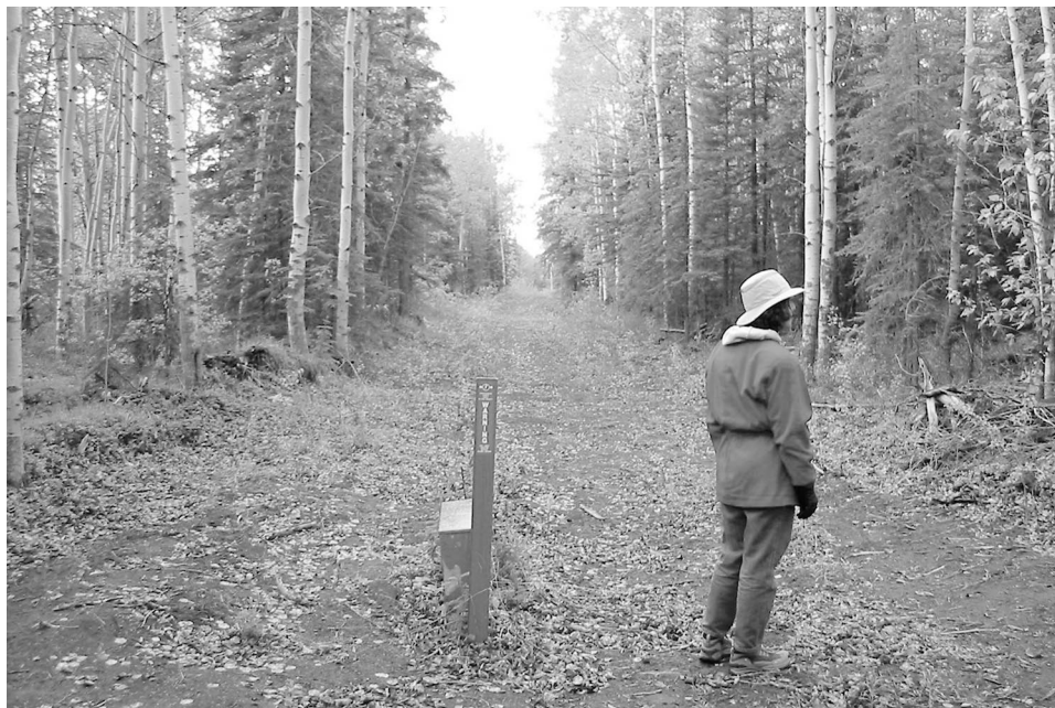
Figure 6: Copper Valley’s Underground Electric Line Crossing Howard Jerue’s Native Allotment (May 2004)
