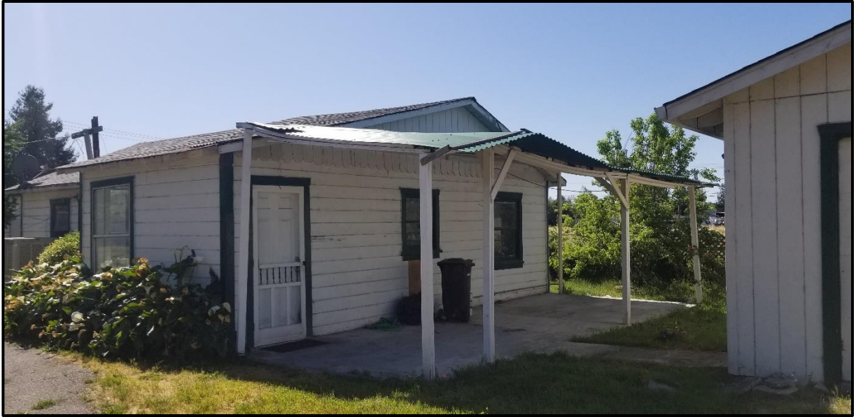
Figure 5. House at 6050 Old Redwood Highway (Map number B). View of north and west side of building.
