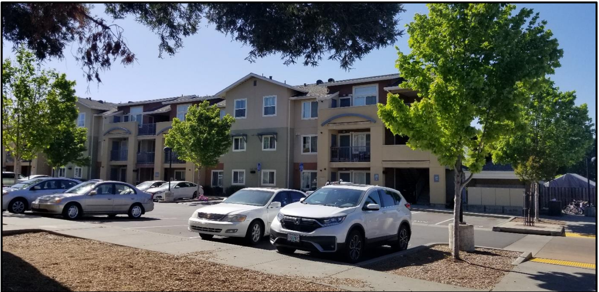
Figure 12. Example of buildings at 100 Kendall Way (Map number 1). View of north side of building.
