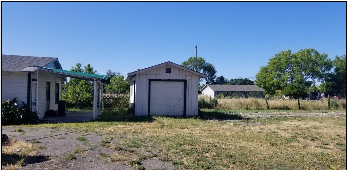
Figure 6. Garage at 6050 Old Redwood Highway (Map number B). View of north side of building.
