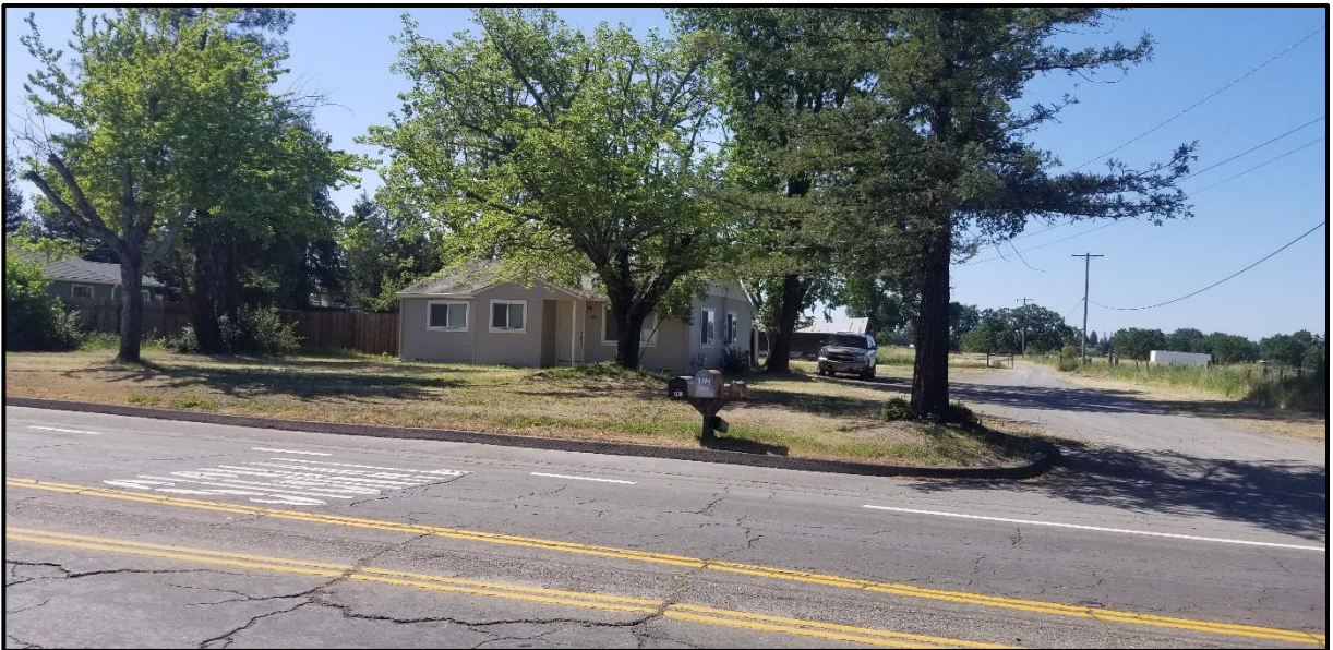
Figure 16. 104 Shiloh Road (Map number 5). View of north and west side of building.
