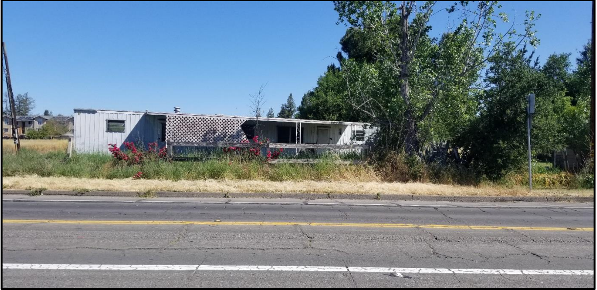
Figure 11. Manufacture home at 6011 Shiloh Road (Map number C). View of south side of building.
