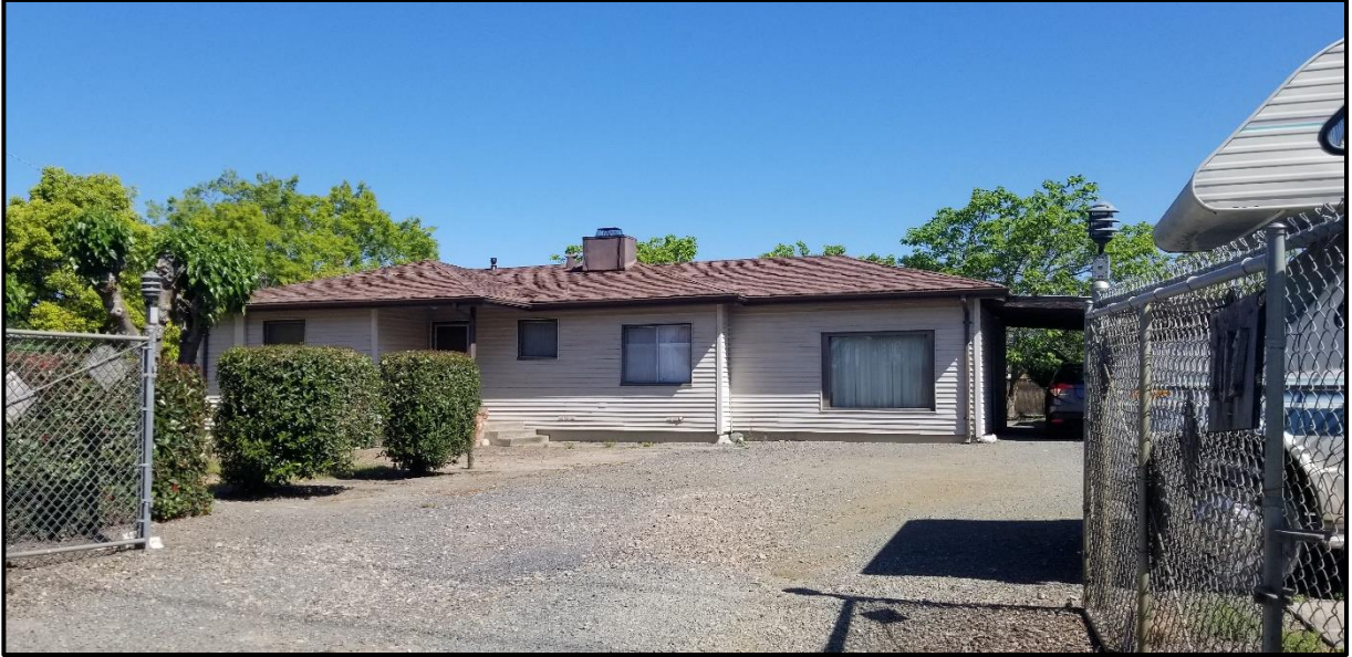
Figure 15. 101 Shiloh Road (Map number 4). View of south side of building.
