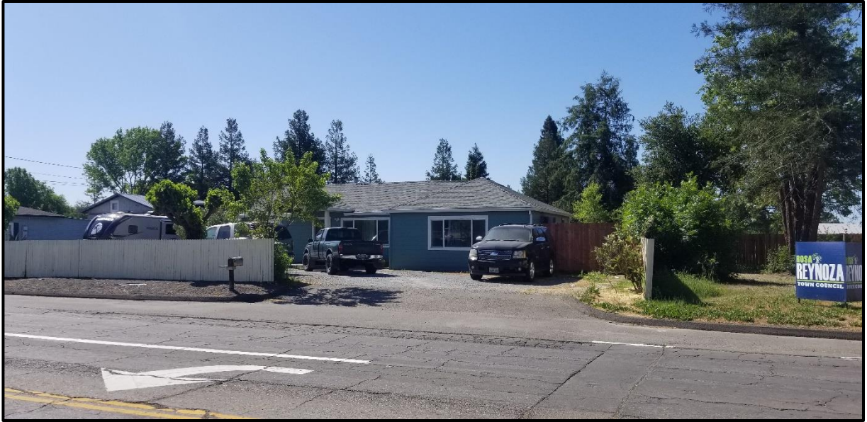
Figure 17. 74 Shiloh Road (Map number 6). View of north side of building.
