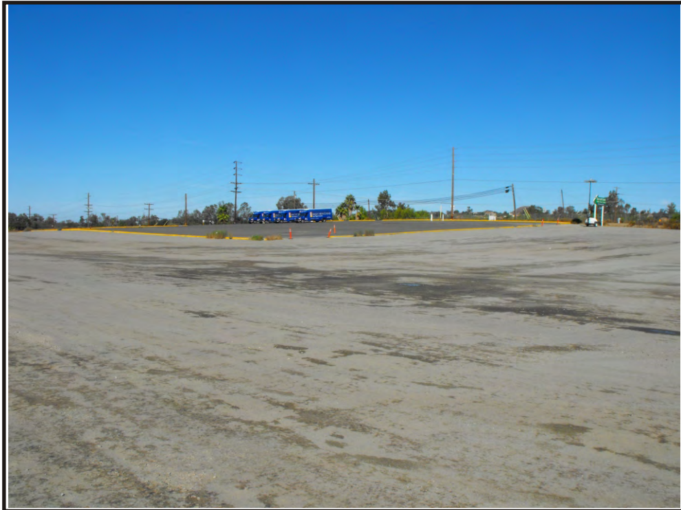
Project Location Overview, View to Northwest (PR-02671-024)
