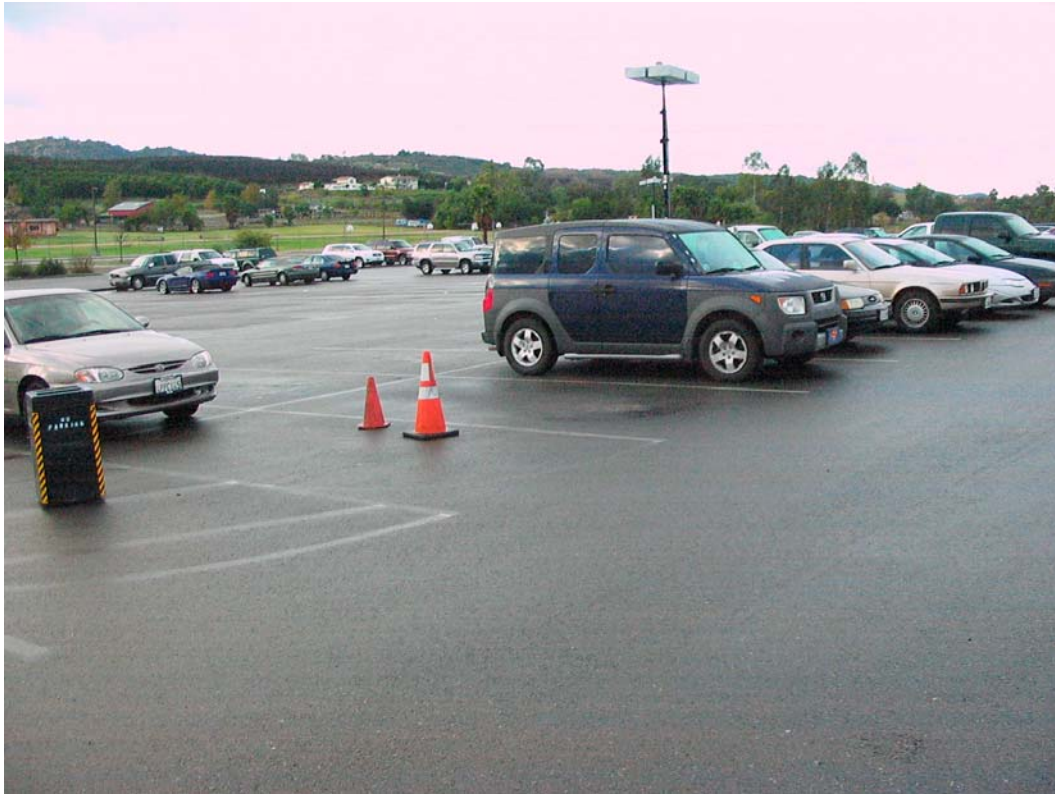
Photograph 5: Asphalt portion of parking lot near northern parcel boundary.
