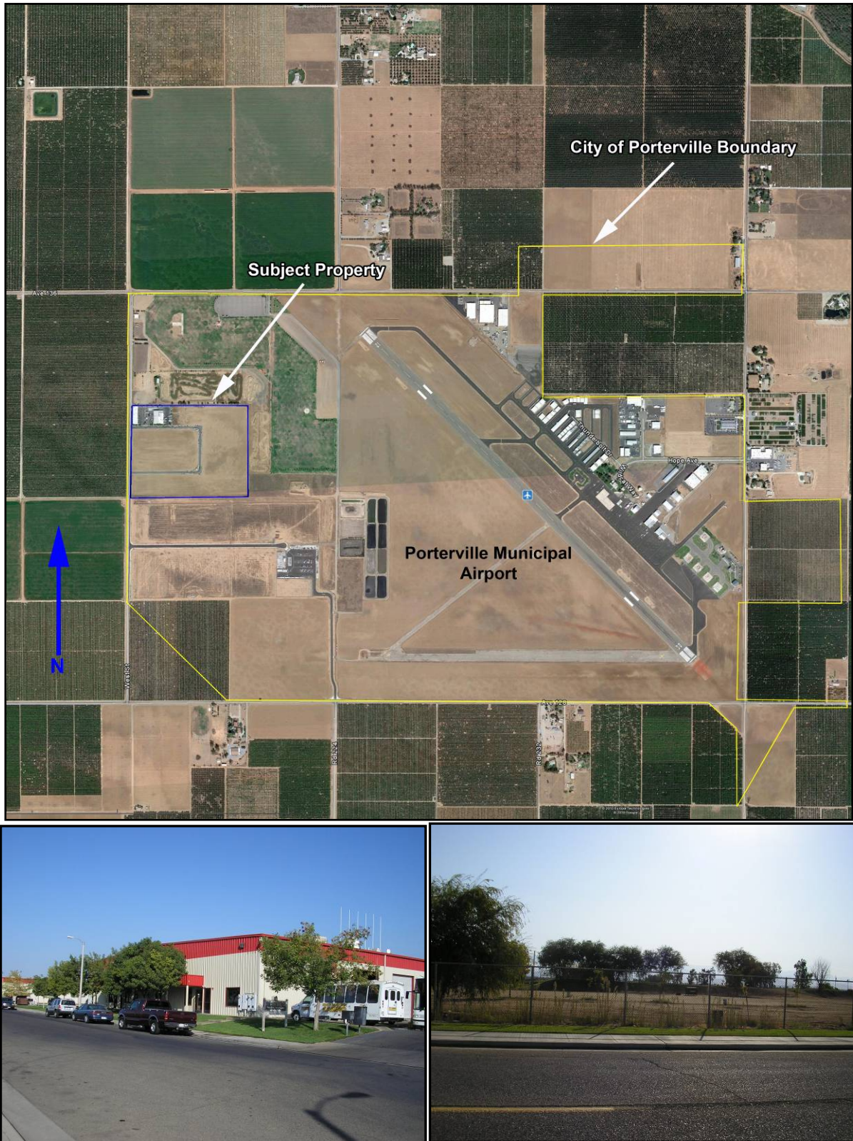
Figure 2-2 Aerial Map and Photos of Site
