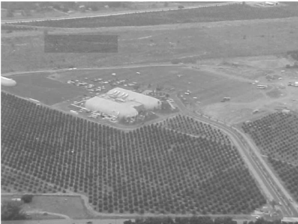
Plate 24: View of Casino Pauma looking southeast.
