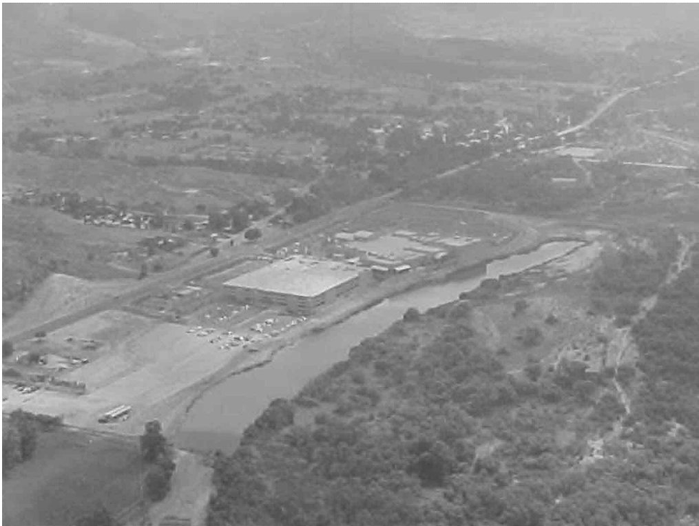
Plate 20: View of the Pala Casino looking northeast. Water feature is the San Luis Rey River.
