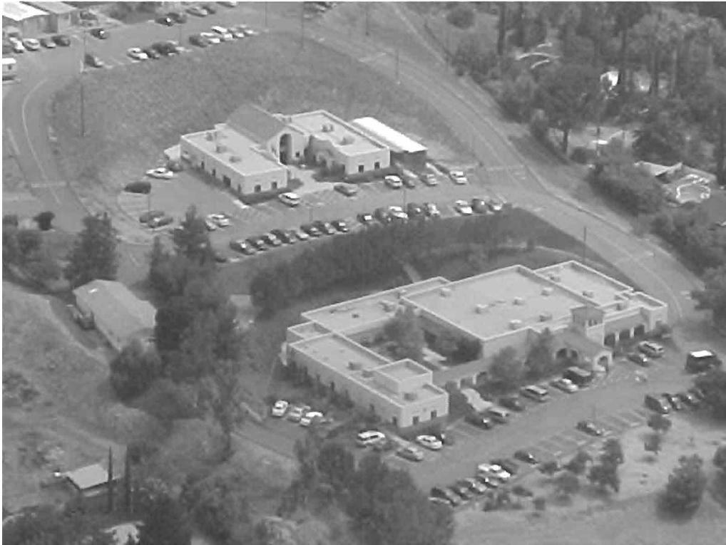
Plate 5: View of the Southern Indian Health Clinic from the southwest.
