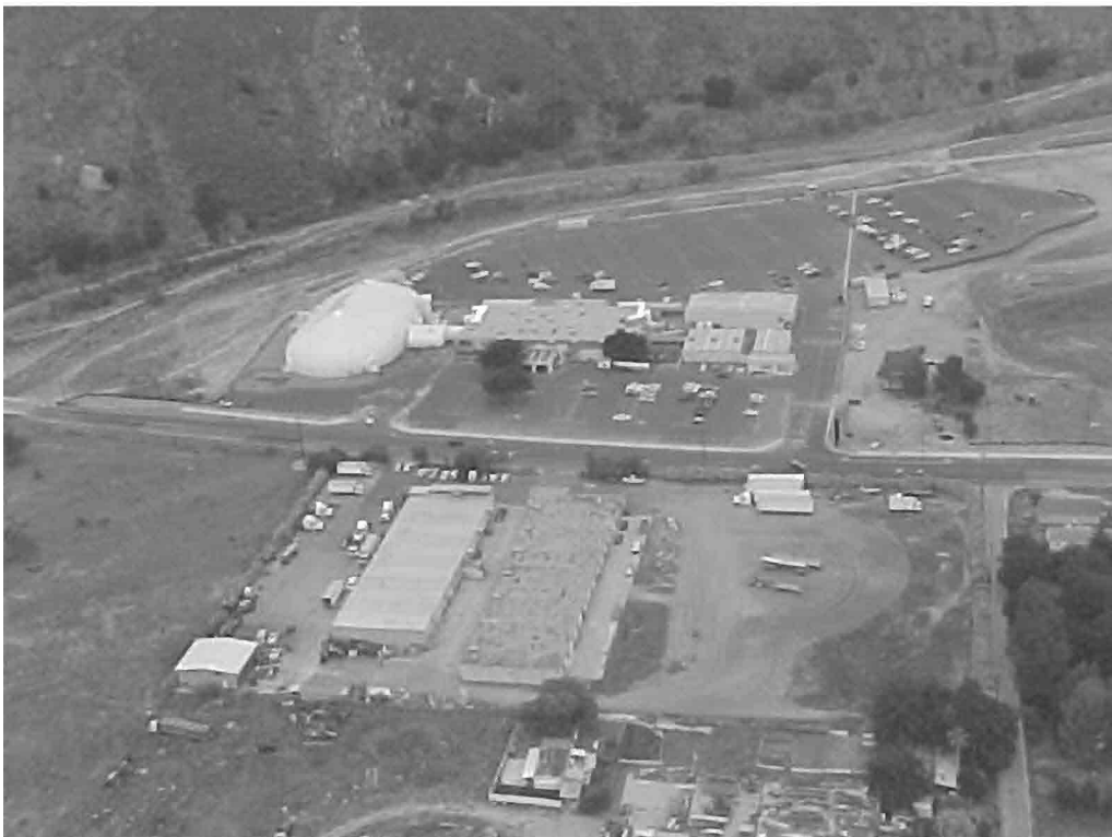
Plate 26: View of the Rincon Casino looking west.
