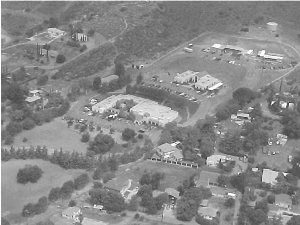
Plate 3: View of Southern Indian Health Clinic Facility on Willows Road, looking northwest.
