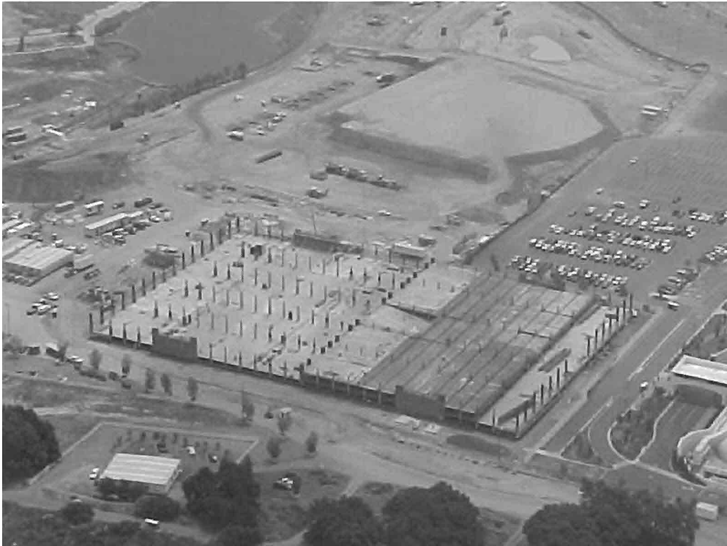
Plate 17: New facilities under construction at the Barona Casino.
