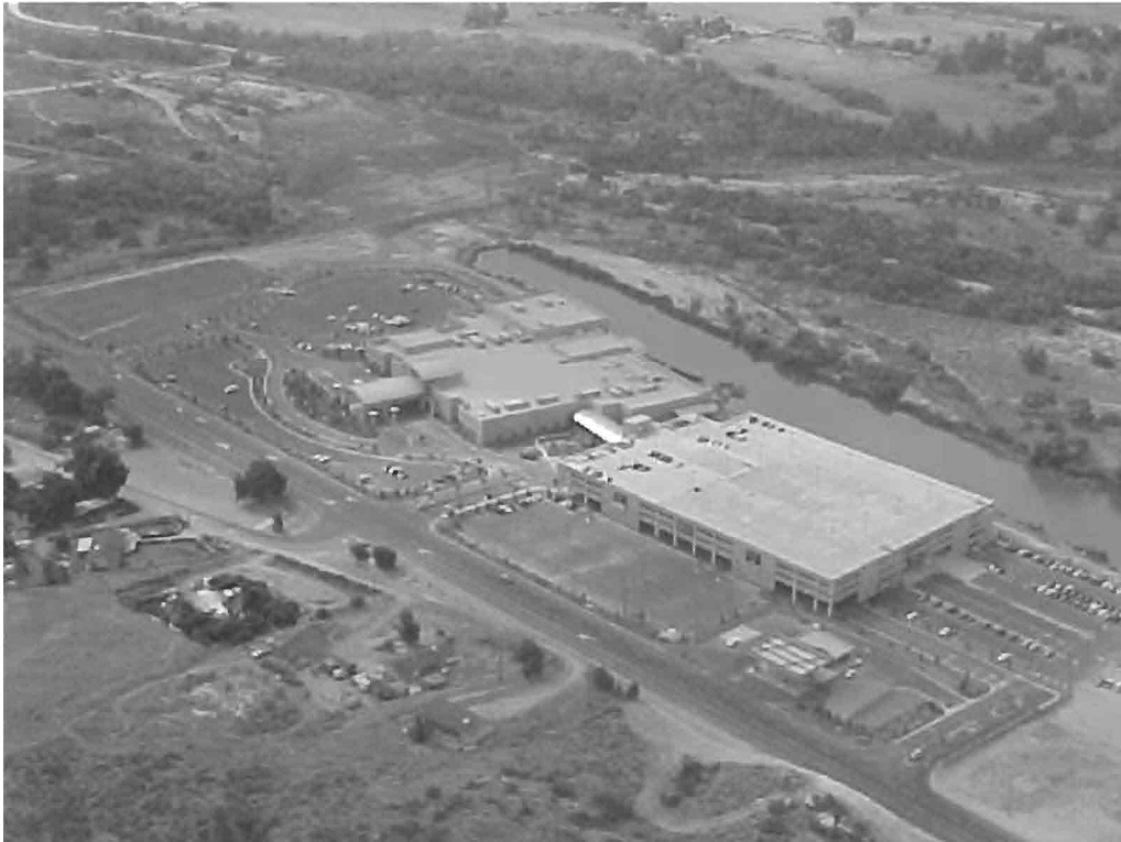
Plate 21: View of the Pala Casino looking southeast.
